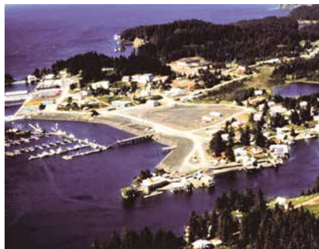
After the earthquake, Seldovia's old waterfront was replaced by a large gravel fill area that remained undeveloped for years.
