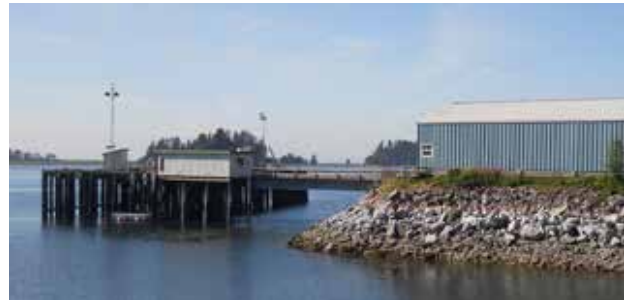
Industrial and marine-oriented land uses are critical to the City.
